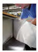
TARABUS floor covering with self-adhesive backing
